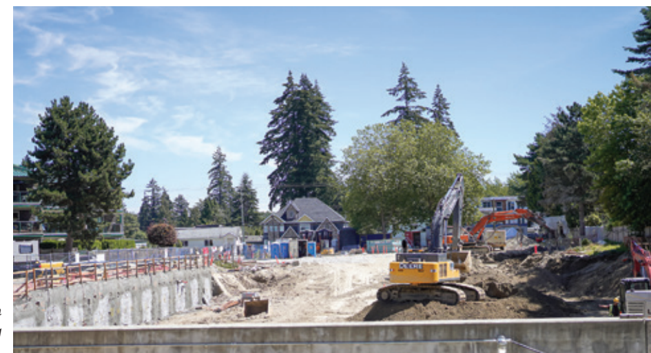
Construction has started on KekinoW’s newest building
