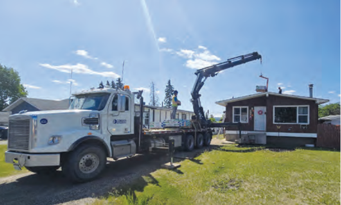
Roof replacement at DCNHS-managed properties
